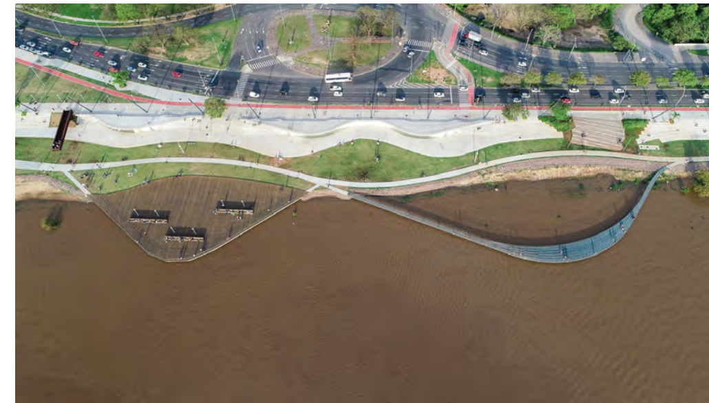
"Guiba Orla Urban Park/ Jaime Lerner Arquitetos Associados," ArchDaily, Accessed December 12 2019, https://www.archdaily.com/907900/guiba-oria-urban-park-jaime-lerner-arquitetos-associados
