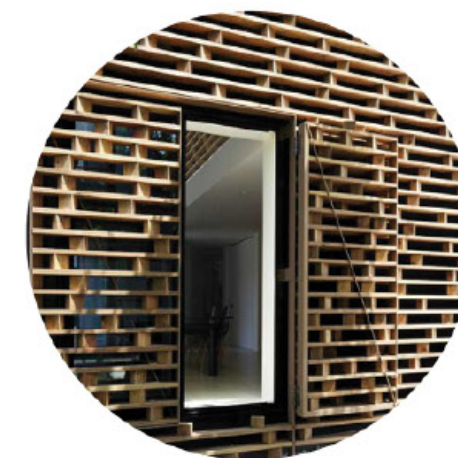
Using wood screen around the openings to create interactive facade for visitors as well as allowing the light in The wood pattern mimicking the form of brick
