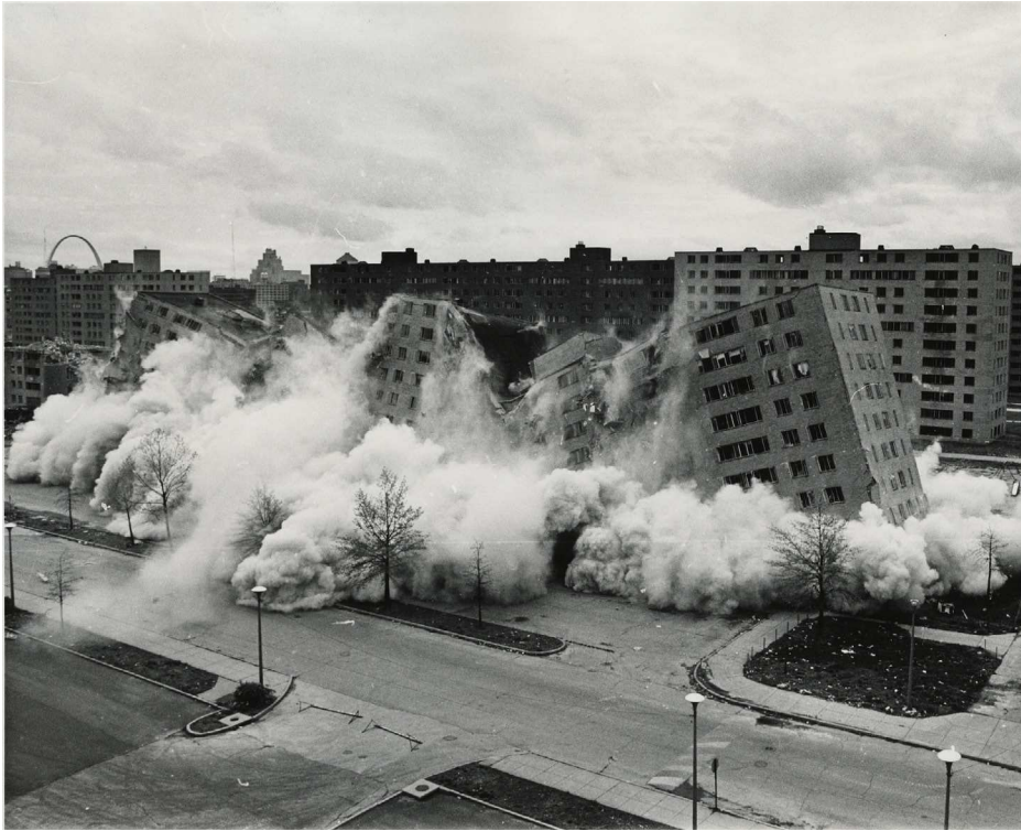
Figure 2 Pruitt-Igoe Apartments, Minoru Yamas, 1954
